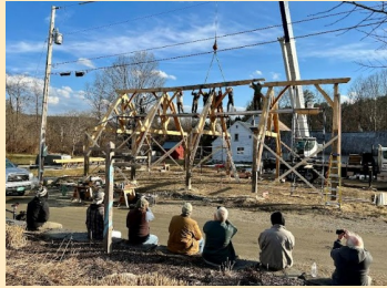
Community members pounding pegs into the timber frame beam.
