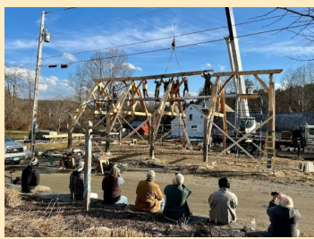
Community members pounding pegs into the timber frame beam.
